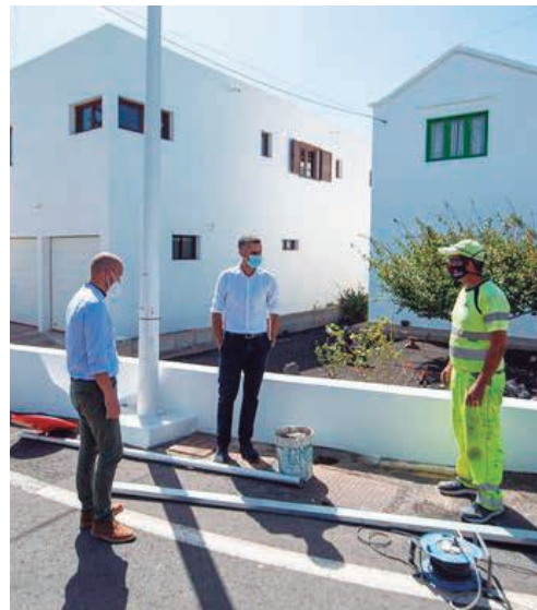
The Town Hall is in the final stages of replacing 186 older lampposts with renewable energy Led bulbs at locations in Playa Honda. These are more economical to run, improve the quality of public lighting and help conserve the environment, according to Public Works Councillor Raúl de León
