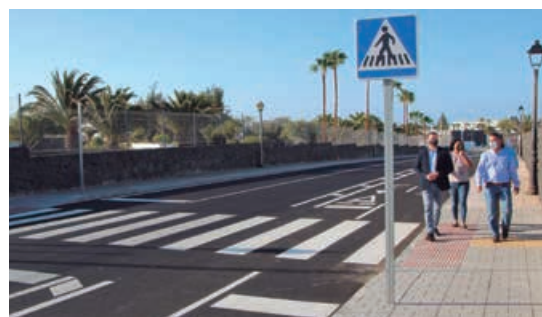
Energy-efficient led lighting installed at Playa Blanca
