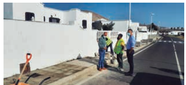
The Town Hall has resurfaced and repaired pavements
