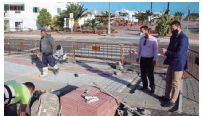
Yaiza has improved accessibility to pavements in the central Avenida Papagayo at Playa Blanca in tandem with works on roads in Costa Papagayo. Calle Molina has been entirely rebuilt with pavements and a bike lane. The Mayor is seen with the Councillor for Public Works Jonatan Lemes
