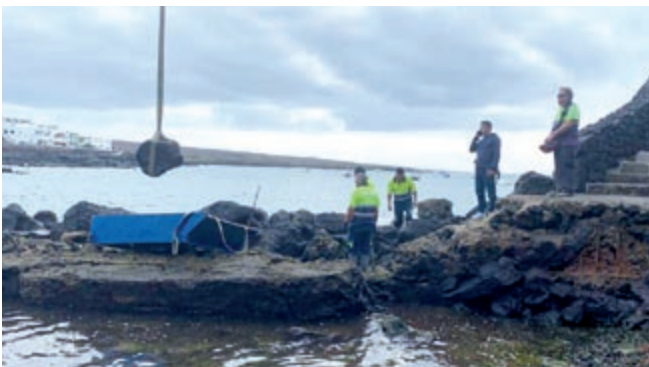
Under an agreement with the Ayuntamiento of Haría the Cabildo Public Works department is repairing the entrance to El Muellito Dock at Punta Mujeres
