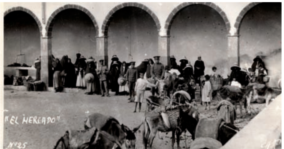
The Recova was the capital's original public market which is still preserved at the rear of the Ayuntamiento and is sometimes used for concerts
